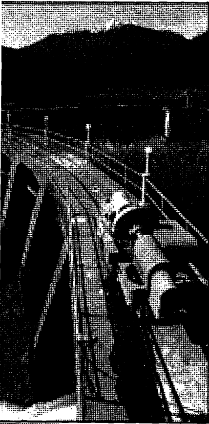
Spillway bridge, Glines Canyon Dam. (Pat O'Hara)
