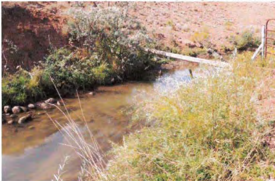
Figure 3-2: Water flow in Deep Creek Canal during the September 18, 2012 site visit.
