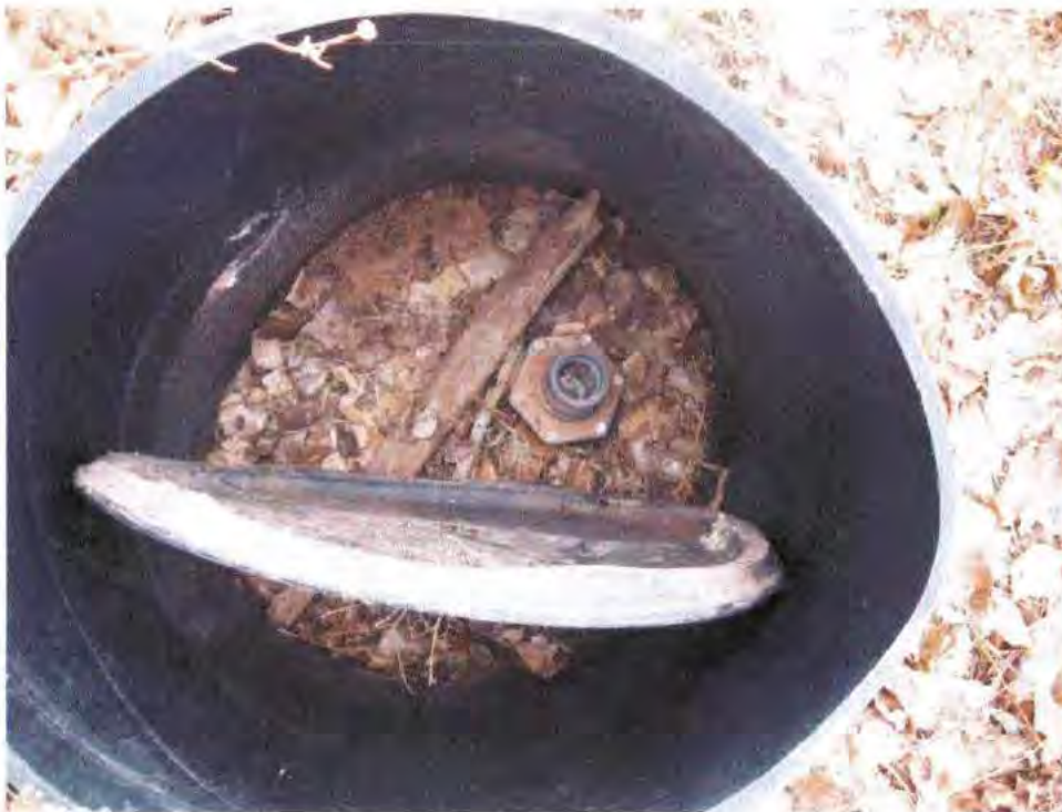
Figure 3-3: Valve housing and hexagonal flange.
