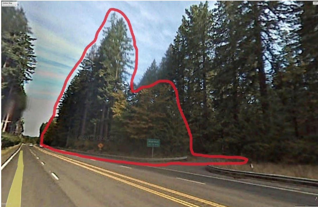
Before Widening – 2008 (2-ER-177)
