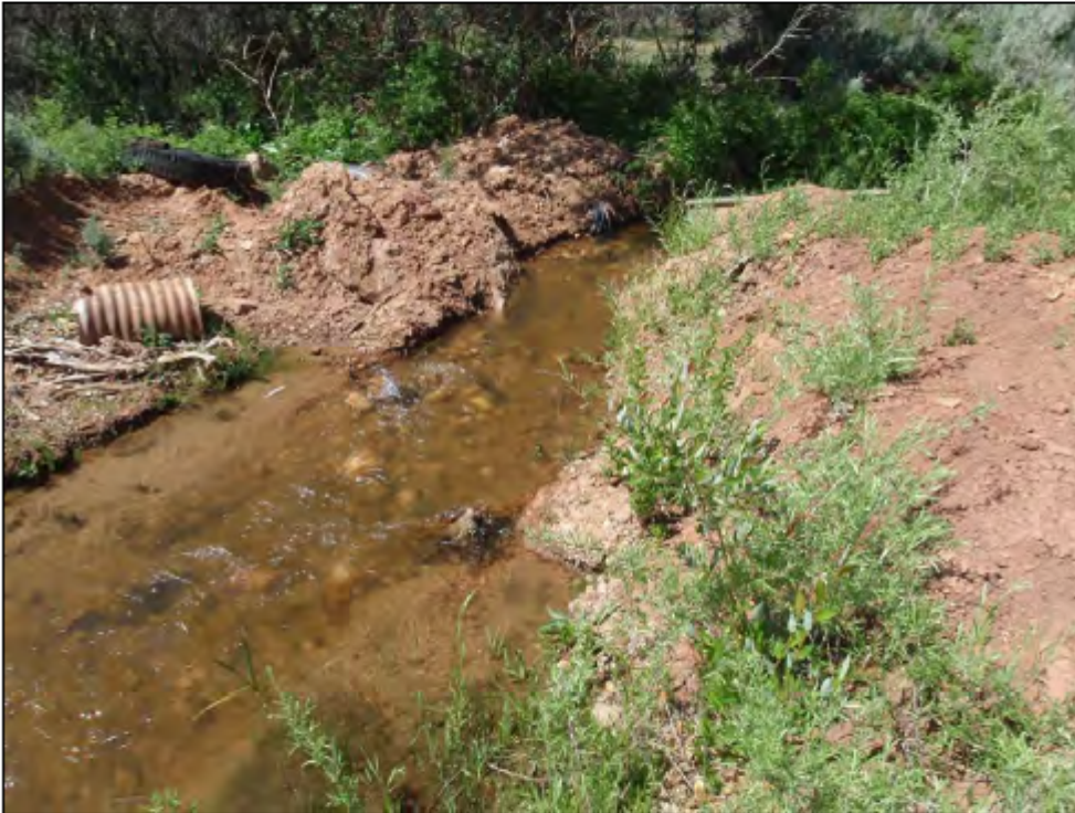
Figure 3: Diversion into Lateral 9 from Deep Creek Canal.
