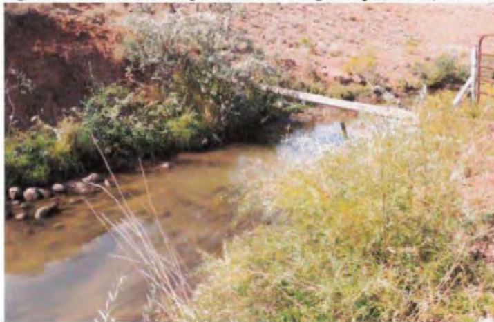
Figure 3-2: Water flow in Deep Creek Canal during the September 18, 2012 site visit.
